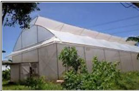
Fasilitas screenhouse dataran rendah
